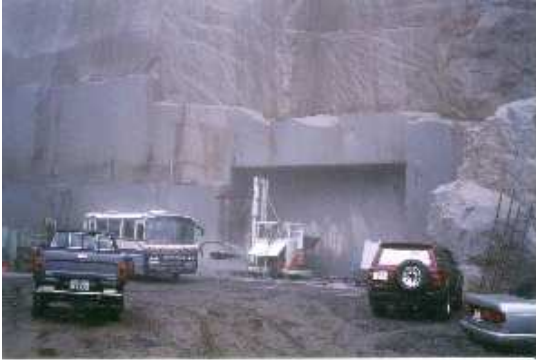
Figure 2. Tunnel excavation in a Japanese quarry by means of waterjet slotting equipment.
