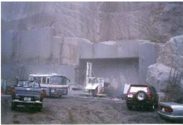
Figure 1. Tunnel excavation in a Japanese quarry by means of waterjet slotting equipment
