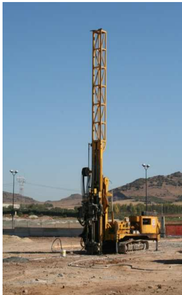
Figure 8. Water injection system: tracked vehicle with lance, pump and control panel
